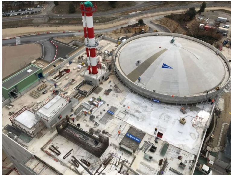
Figure 21 – State of construction in May 2017
