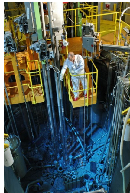
View of the reactor pool, above the pile block
